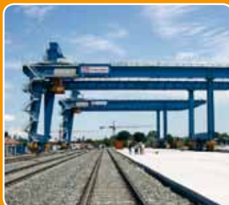
Rail mounted gantry crane, RMG.
