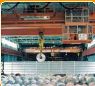
Rail mounted gantry crane, RMG.
