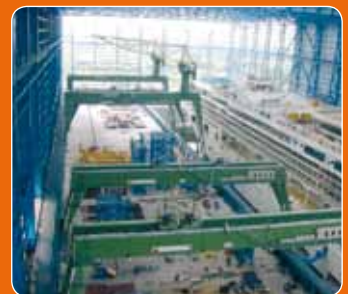
11- Shipyard gantry crane.
