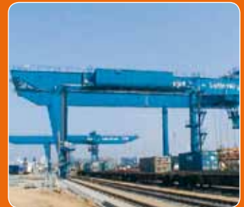
8- Container portal crane.
