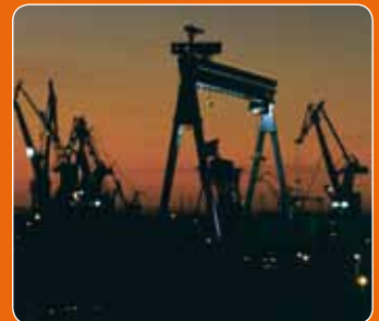
10- Goliath crane for shipyard.
