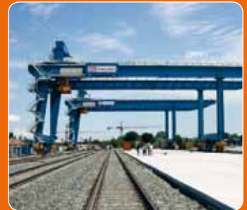
7- Rail mounted gantry crane, RMG.
